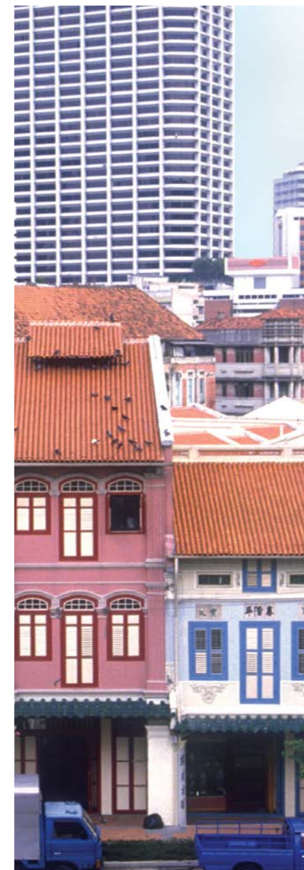
Shophouses in the Tanjong Pagar area were among the first heritage structures to be restored in 1987. MITA collection, courtesy of National Archives of Singapore.
