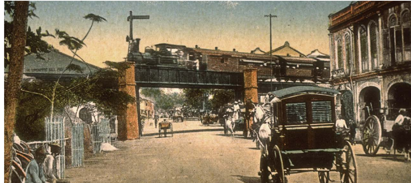
The overhead link between the two buildings that comprise Orchard Gateway today harkens back to the railway bridge (1903–1932) that was once found in Orchard Road. It is a reminder that we can find resemblances of the past in Orchard Road's present if we look hard enough – perhaps some consolation to Tan Wee Him (see quote below) and his like-minded peers. Courtesy of National Archives of Singapore.
